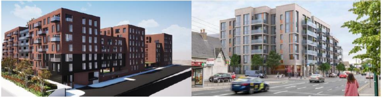
Fig. 1 – Permitted developments in the immediate vicinity – Santry Place, 7 storeys (on the left) and Swiss Cottage, 7 storeys (on the right)
